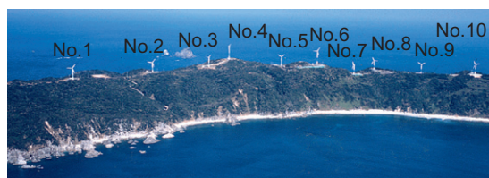
Fig. 15. Actual wind turbine installation positions of the Noma cape wind power plant in the Kagoshima prefecture.
